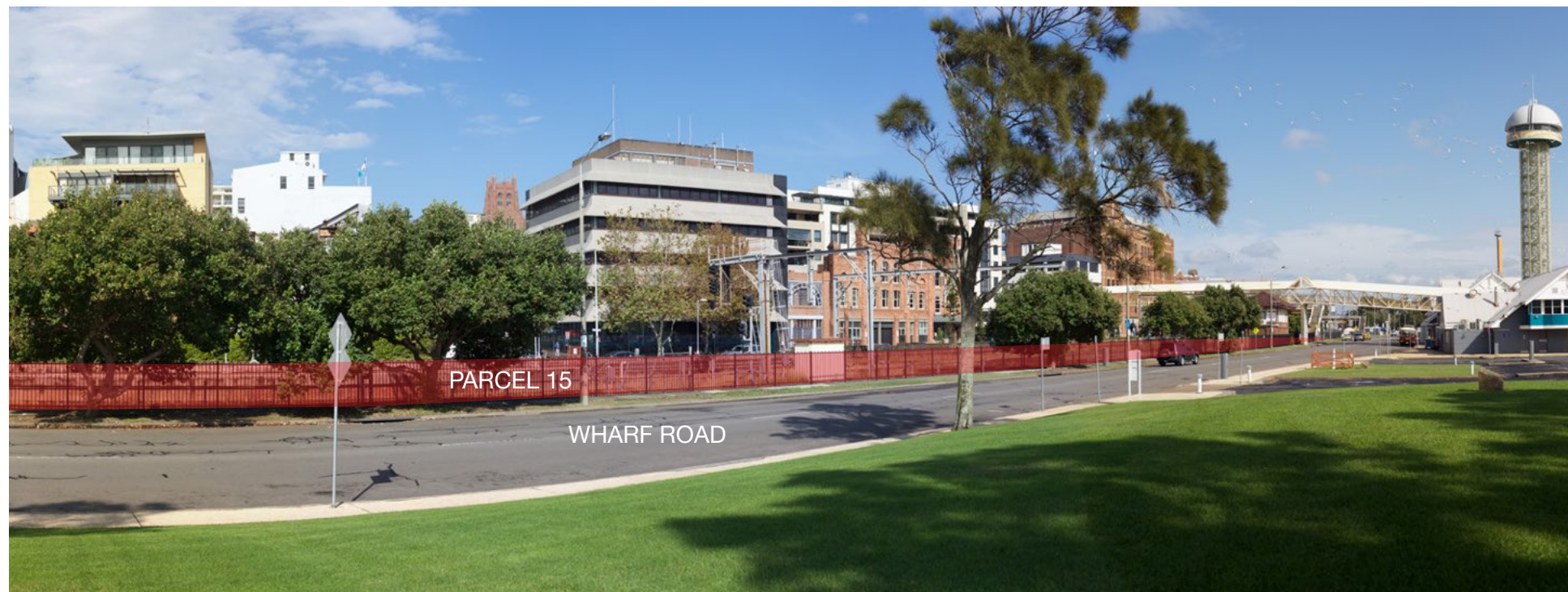
Viewpoint 08. View from Wharf Road in a generally South West direction
