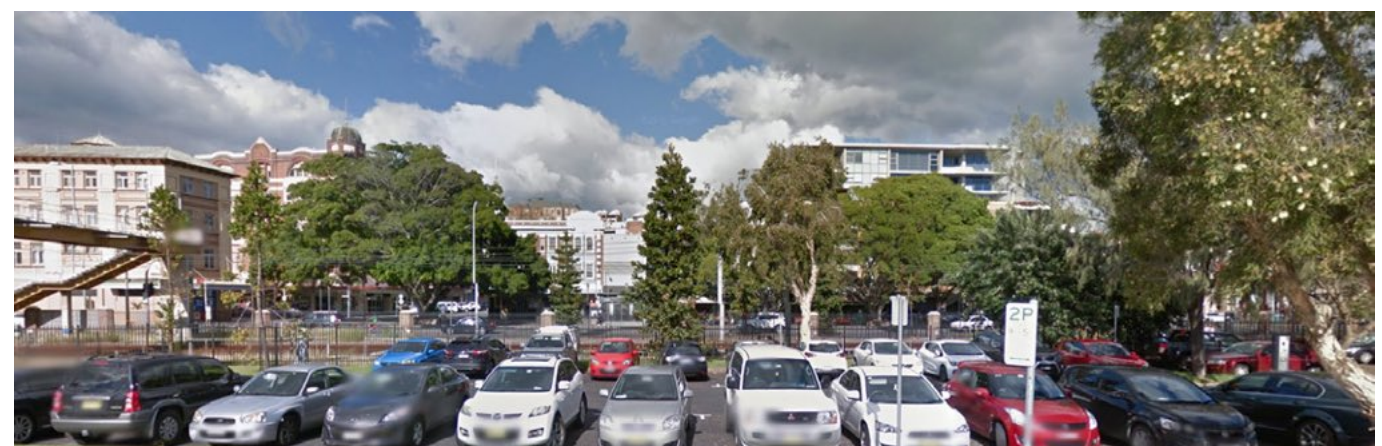
Image 15. View from Wharf Road illustrating existing street trees fragmenting views from buildings along Hunter St
