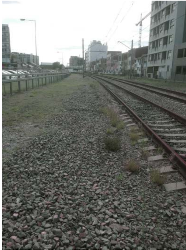
Plate 1 Existing rail within the site
